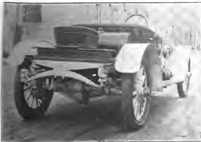
Showing rear axle of Collins Axle Mfg. Co., of Pittsburgh
